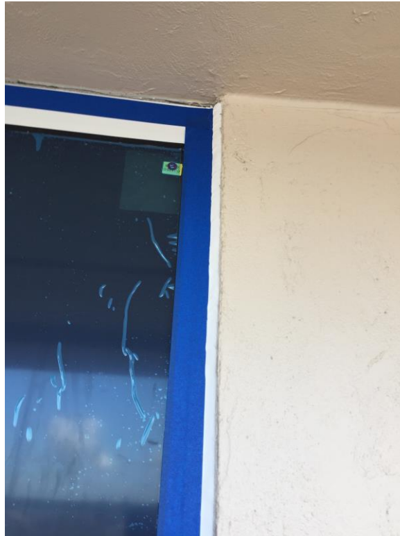
Picture 5: Typical caulking application
