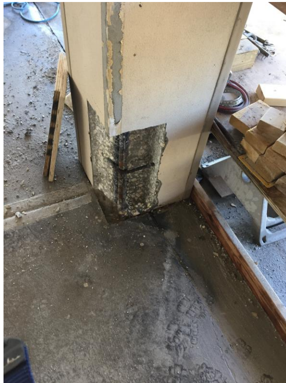
Picture 4: Approved column excavation
