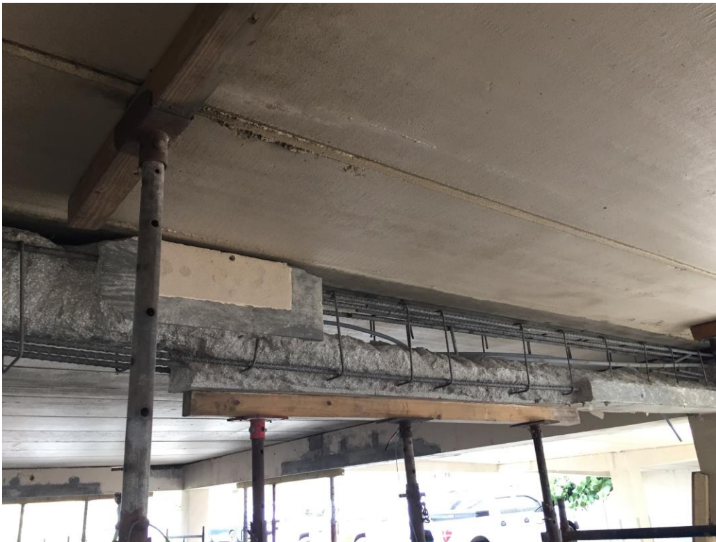
Picture 2: Approved beam excavation
