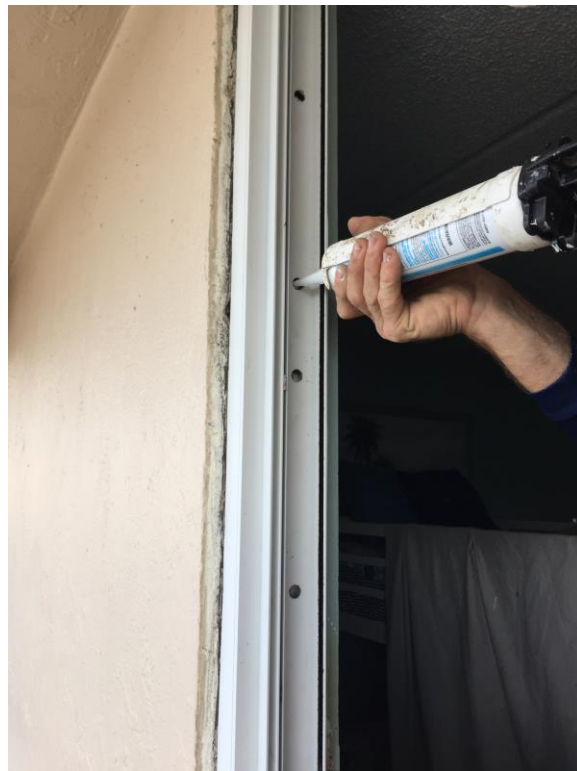
Picture 6: In-progress caulking of fastener heads
