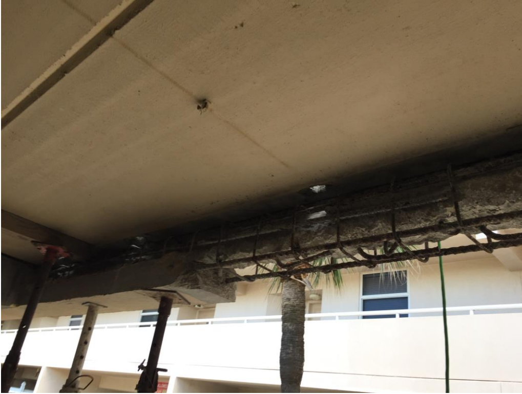
Picture 1: Approved beam excavation
