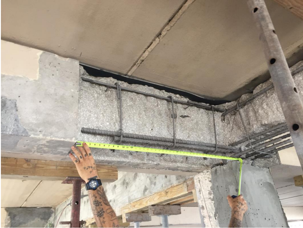
Picture 3: Approved beam excavation
